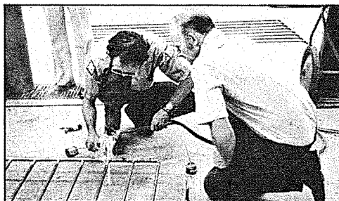
Practical classes, such as this "How to Plan, Construct and Install a Solar Waterheating Unit" course, are offered under the Adult Non-credit and Institutional Credit Programs of Continuing Education.
